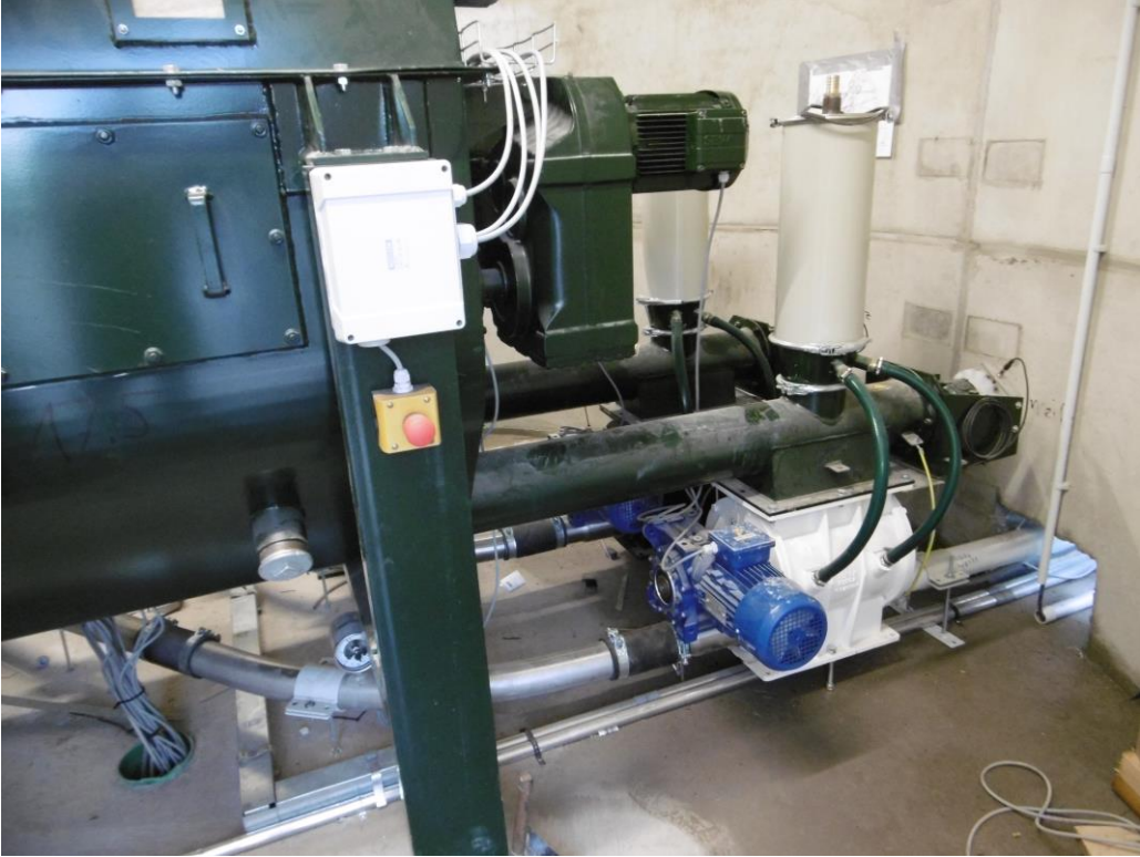
2 separate Dosing lines: To burner "white" line To burner "black" line
