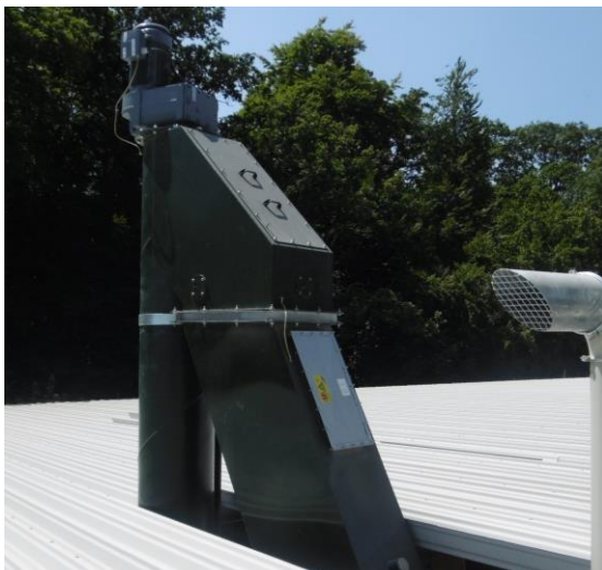
Feeding chute with blow-out disc
