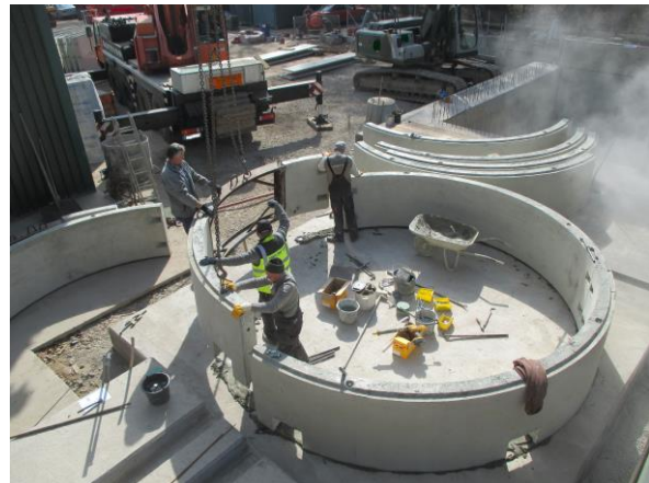
Erection of fuel silo
