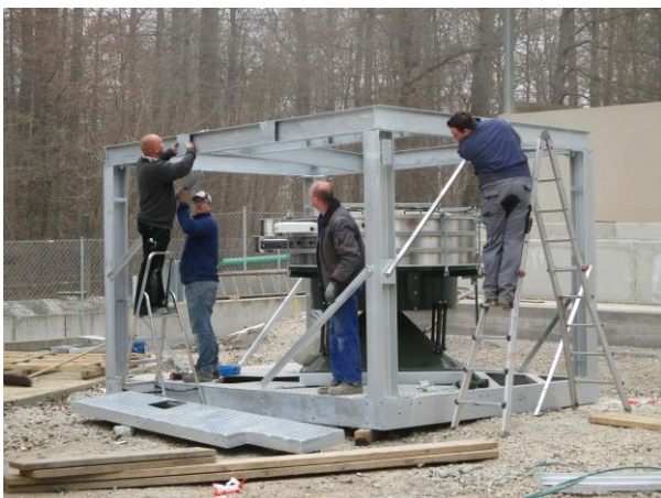
Preassembly of one module Of processing system
