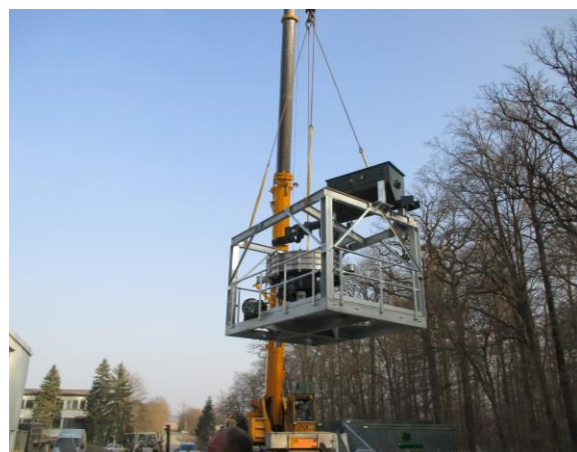
complete module gets lifted and connected to the plant
