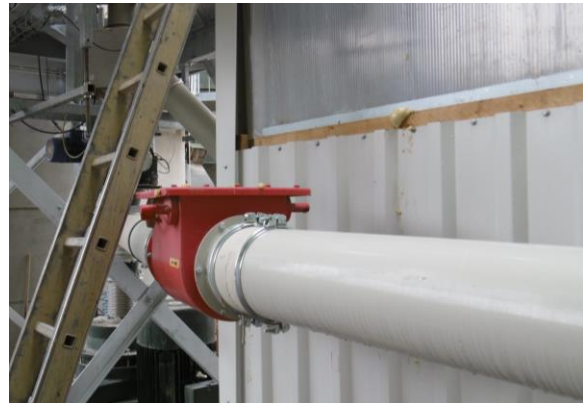
Air inlet tube with flame trap
